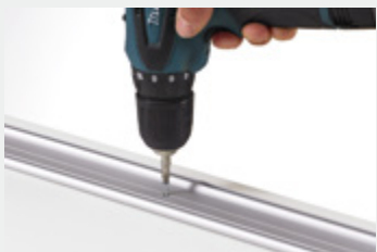
Fix the profile with screws
