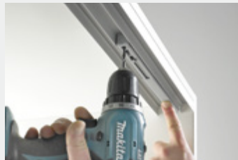
Fix the damper
